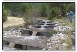
hydraulic modeling of water depths and velocities. The hydraulic model also evaluated the passage channel stability. Our engineers also conducted reservoir routing analysis to specify critical design element invert elevations that control flow distributions to the reservoir outlets and the fishway entrance through the range of design flows.
